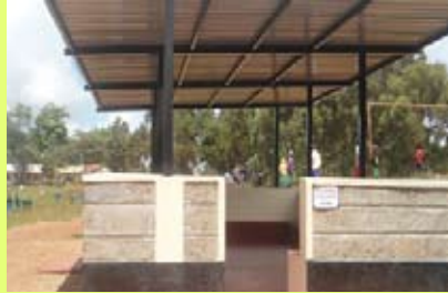
Playing shed for Kyangoma Special Needs School
