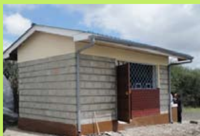
New Kitchen and Store for Kanaani Primary School
