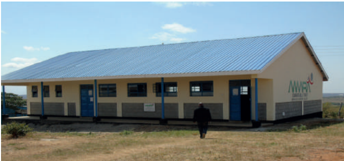
Completed dormitory building
